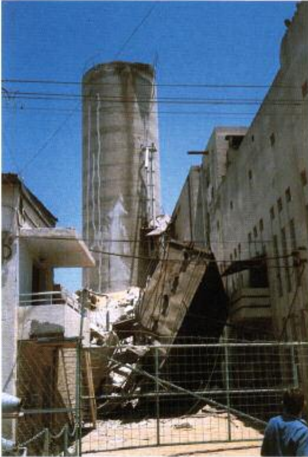
Undamaged silo and debris of collapsed silo
