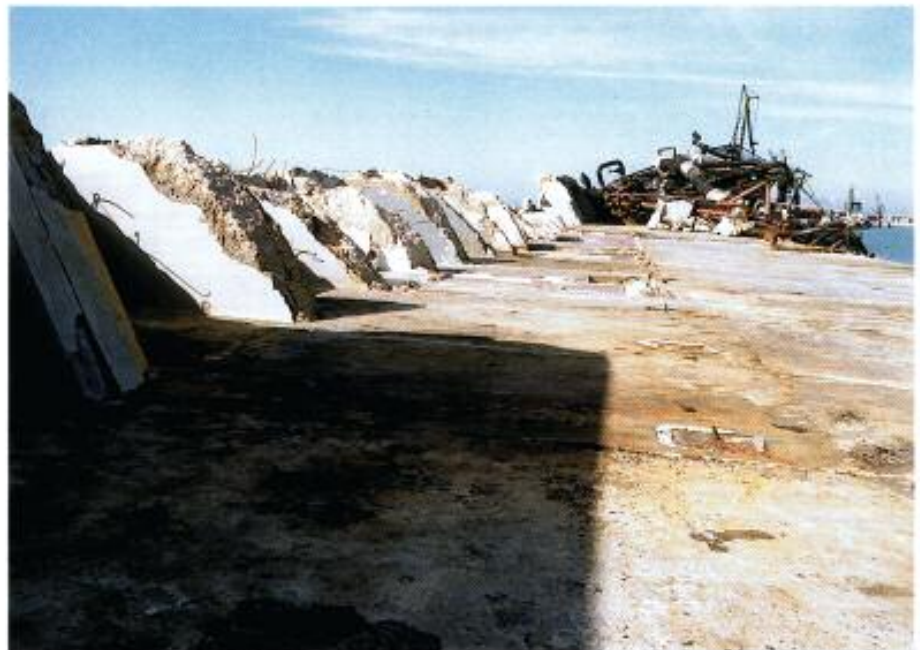
Fig. No. 224 The top of the breakwater and the damaged wavebreaker can be seen to the left, with destroyed equipment in the background
